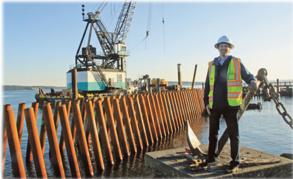
Image: Port Engineer Matt Klontz Oversees Reconstruction of the Point Hudson Jetty – Summer 2023.
