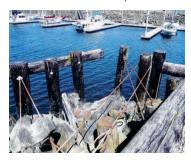
The project involves the total demolition and replacement of the Point Hudson Jetty. The jetty structure, built in 1934, has reached the end of its useful life and is at high risk of catastrophic failure if not replaced. Replacement of the breakwater ensures that the public's substantial existing investment in the Point Hudson Marina remains intact and ready to serve the public. Design and permitting will continue in 2017; construction is now scheduled to begin in 2018.
