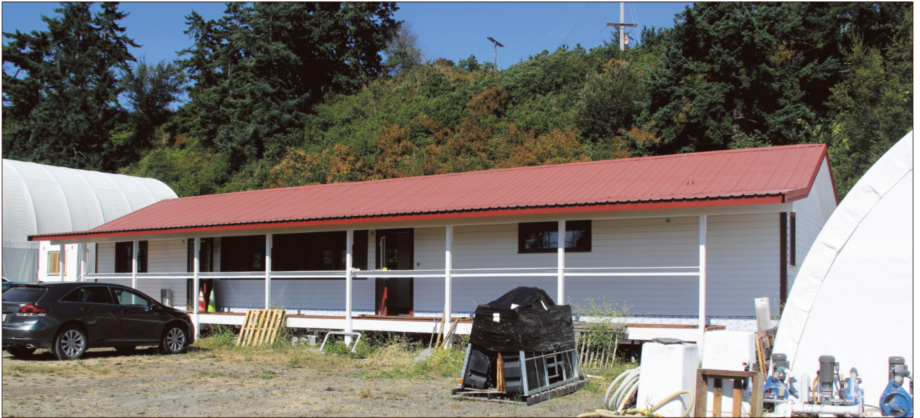
This old Coast Guard building has been completely refurbished by Port staff and now becomes the new expanded moorage office at the Boat Haven Marina.
