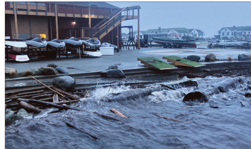
Flooding at the Northwest Maritime Center in downtown Port Townsend was narrowly averted on Dec. 27, 2022, but continued sea level rise is likely.
