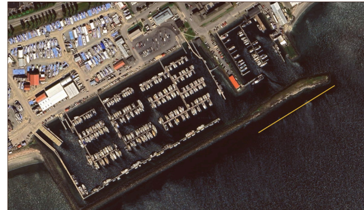
About 550 feet of the Boat Haven Marina breakwater (yellow line) was built in the mid-1930s and is failing. The Port expects to extensively rebuild that section with heavily leveraged IDD funds, hopefully starting this summer.
