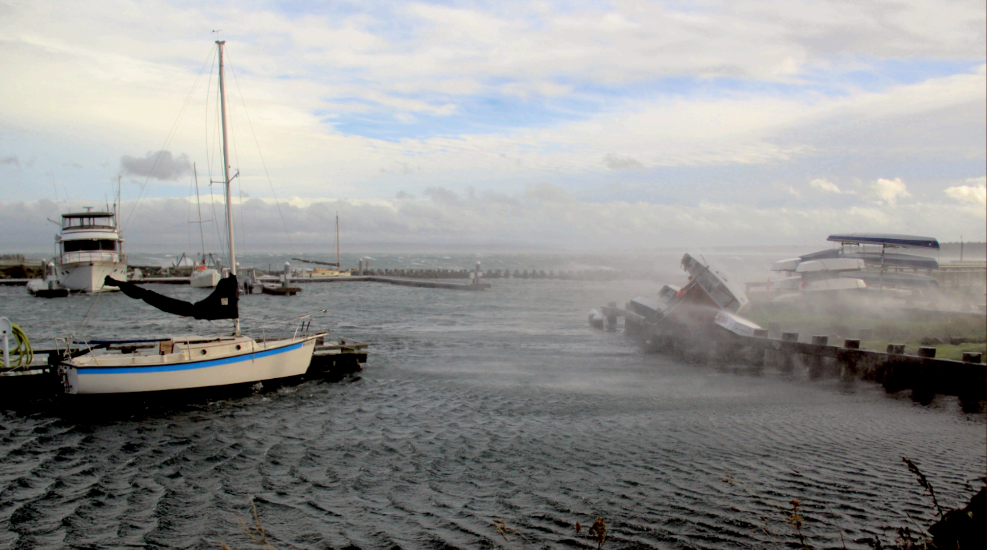
The combination of king tides and winter winds blew through the Point Hudson Marina before the old jetties were replaced, starting in 2022.
