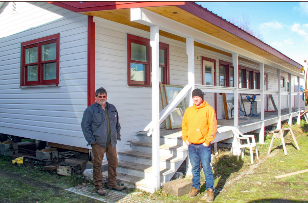
The Port recycled the old U.S. Coast Guard building, which had been hauled off Benedict Spit years ago, into a completely rebuilt Boat Haven Moorage office, which was moved to its new location in the middle of the boatyard in early 2024. Much of the work was done by the Port's maintenance staff, including Dave Johnson, left, and Chris Sparks.
