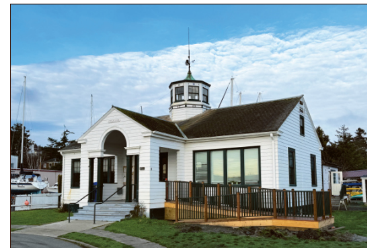
The Cupola House at Point Hudson is probably one of the most architecturally unique buildings in the Port's portfolio. Since built in 1935, it has been home to quarantine station administrative staff, the U.S. Coast Guard, the Navy, the Army, private tenants and now, since mid-2024, the Port's engineering and Point Hudson Marina & RV Park staff.
