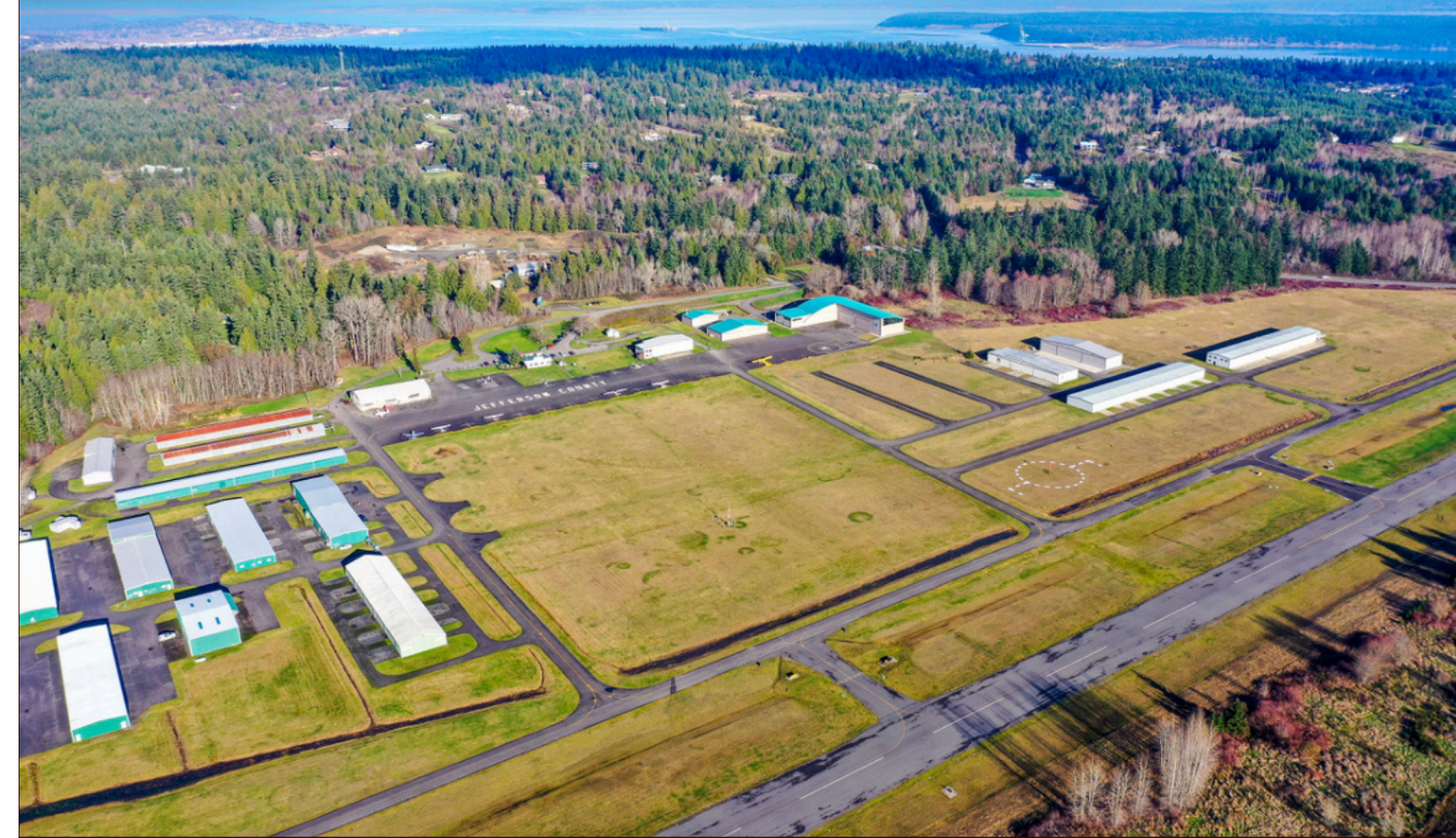
IDD funds played a small but significant role in the rebuild of the Jefferson County International Airport's runway, with almost all of the outside funding coming from the Federal Aviation Administration. Photo by Jim Pivarnik
