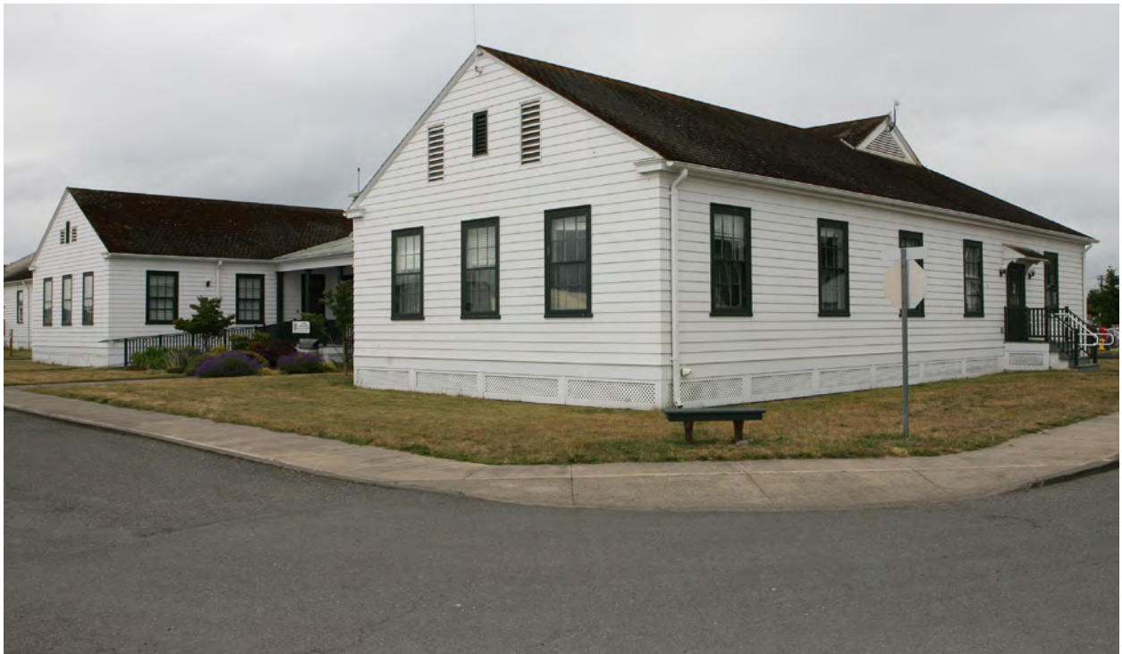
Top: West facade of Hospital, July 2020. Bottom: NE corner of same, July 2020.
