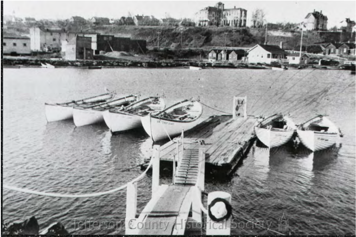
1939 view looking NW across the Point Hudson marina basin. The Pilots Cottage is visible but the Sail Loft and the two buildings south of it have not yet been built. The former Marine Hospital is seen on the bluff. Source: Jefferson County Historical Society. Image ID 2004.117.384. *PENDING PERMISSIONS*
