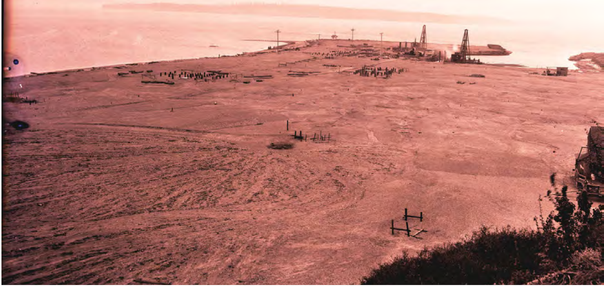
August 1934 view looking south at Point Hudson, showing foundation piles for future buildings and dredging of the marina. Source: Jefferson County Historical Society, image ID 1995.379.7 *PENDING PERMISSIONS*
