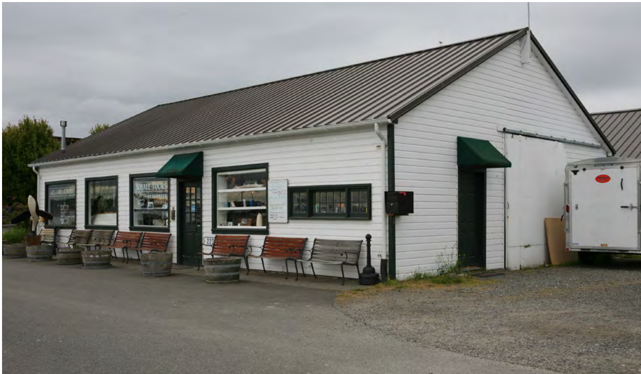
Top: SW corner, July 2020. Bottom: NE corner, July 2020.
