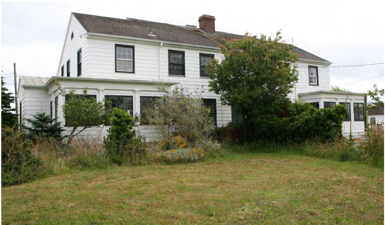
Top: NE corner of Duplex, July 2020. Bottom: NW corner of Duplex, July 2020.
