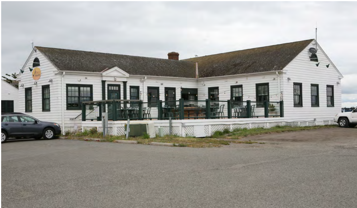
Top: East facade, July 2020. Bottom: West and south facades, July 2020.
