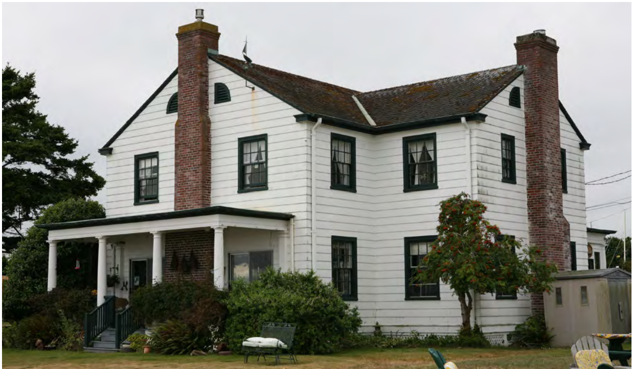
Top: SW corner of bed & breakfast, July 2020. Bottom: NE corner of bed & breakfast, July 2020.
