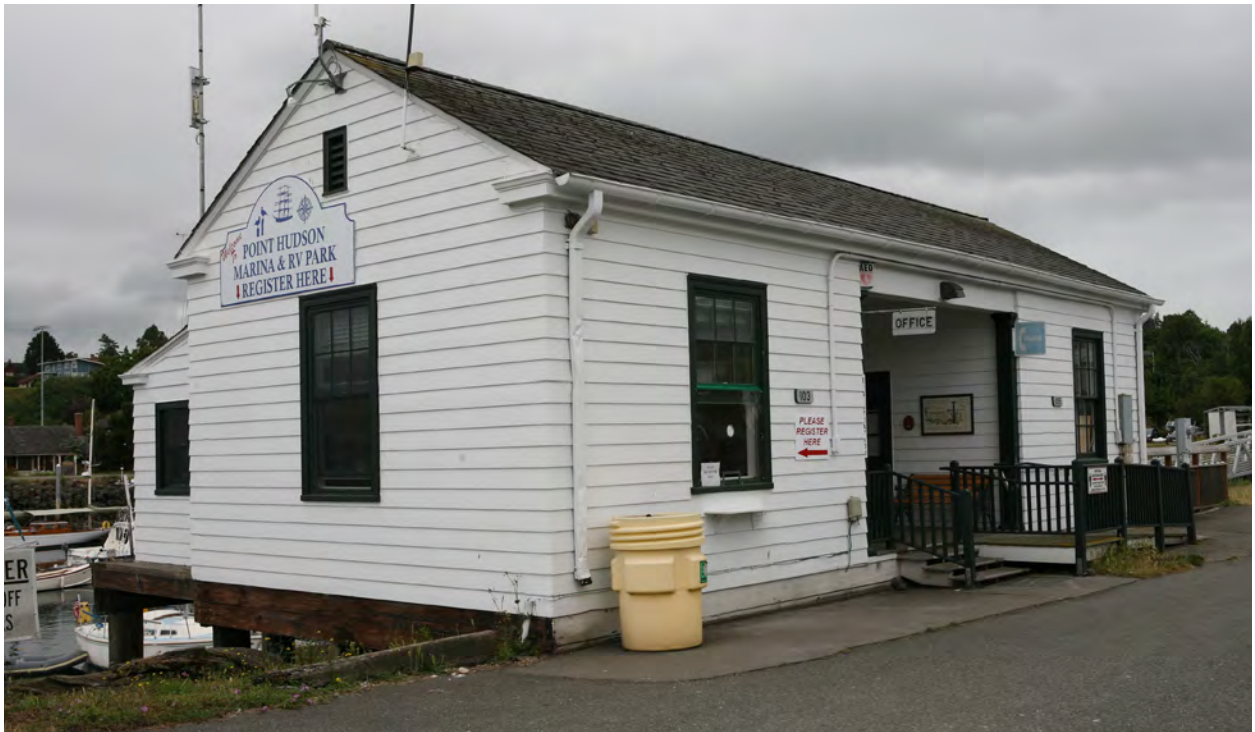
Top: West facade, July 2020. Bottom: SE corner, July 2020.
