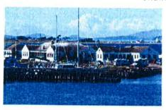
The Point Hudson Administration Building, like others at Point Hudson, rests on creosote-treated pilings and contains creosote-treated floorboards. The 2005 renovation included installation of vapor barrier sheathing and mechanical ventilation to mitigate the creosote odor. These measures have been successful to a large degree, but have not fully solved the ongoing odor issues. Resolving this issue is key to
