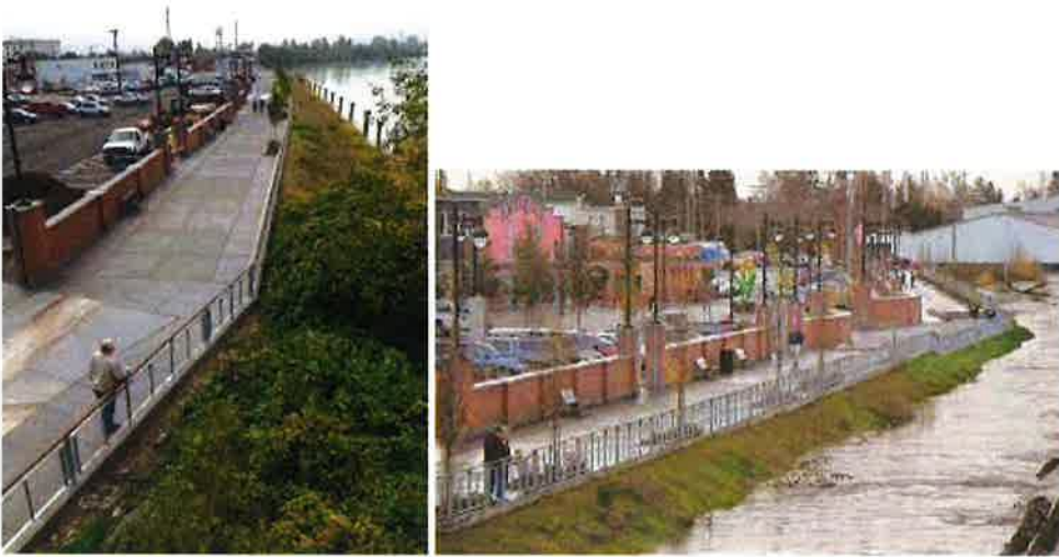
Photos of Mount Vernon's flood protection structure/walkway along the Skagit River.
