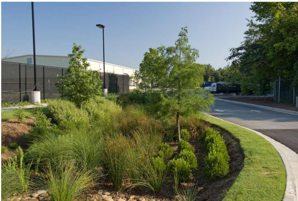
Example of Bioretention Cell
