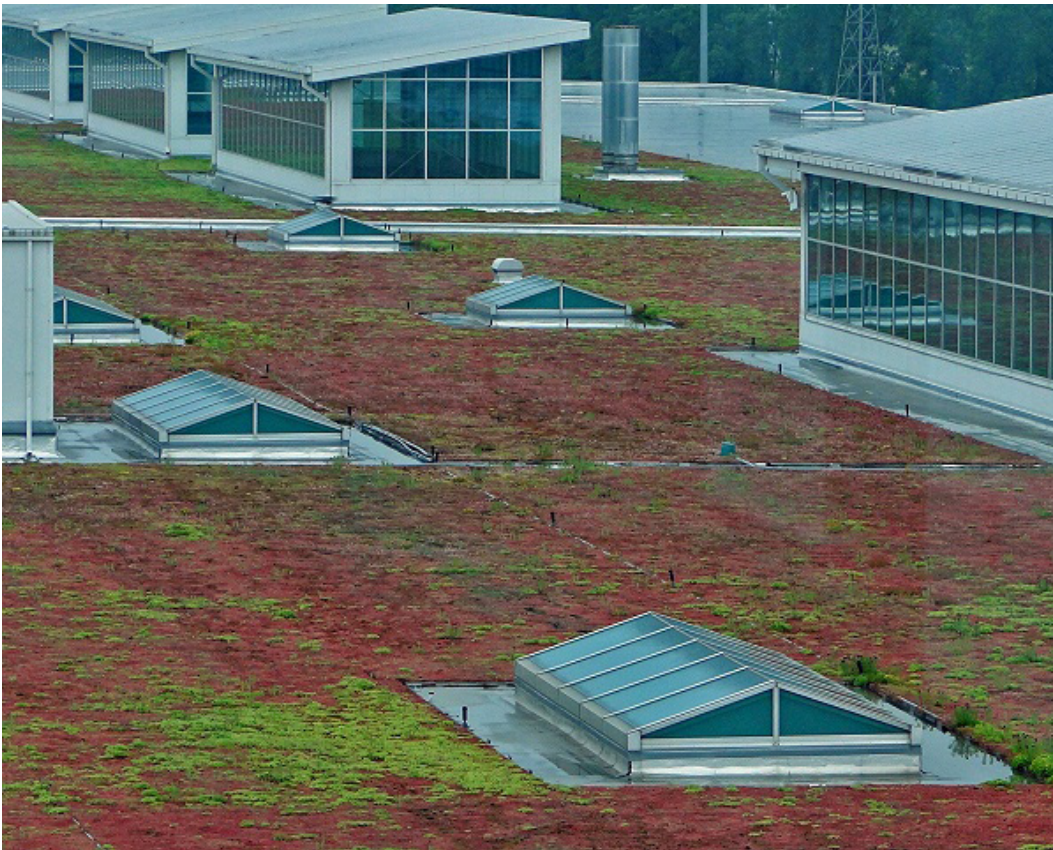
Example of Green Roof
