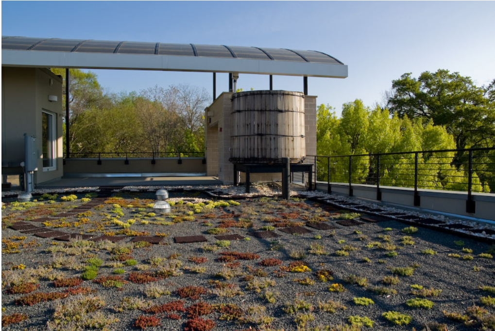
Example of Green Roof and Rainwater Capture Cistern
