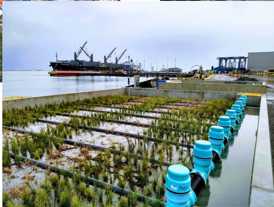
Biofiltration system in Port Angeles, designed by Kennedy Jenks
