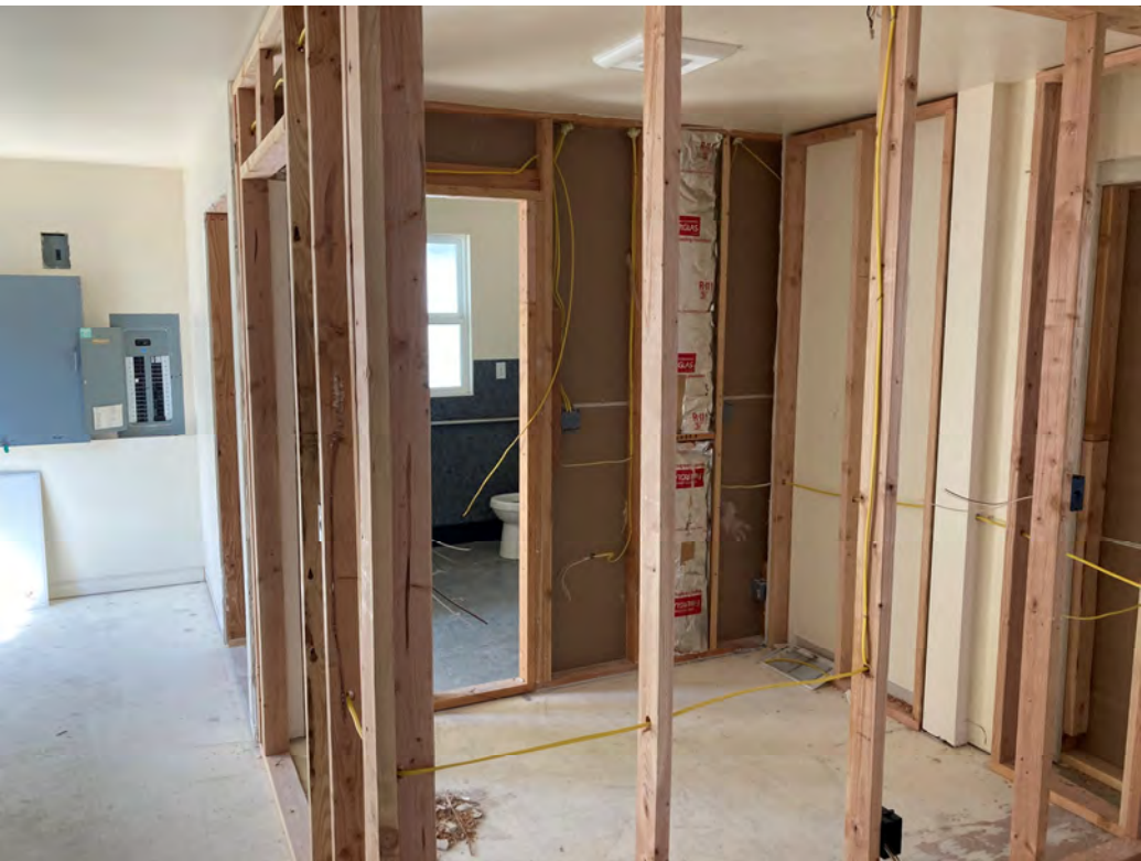
Framing and rough electrical for Second Restroom.
