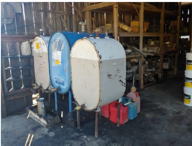
5. Petroleum ASTs in Lumber Shed
