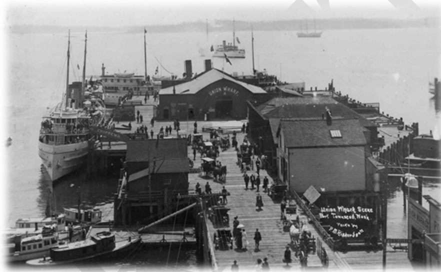
Old Union Wharf – Port Townsend, WA
