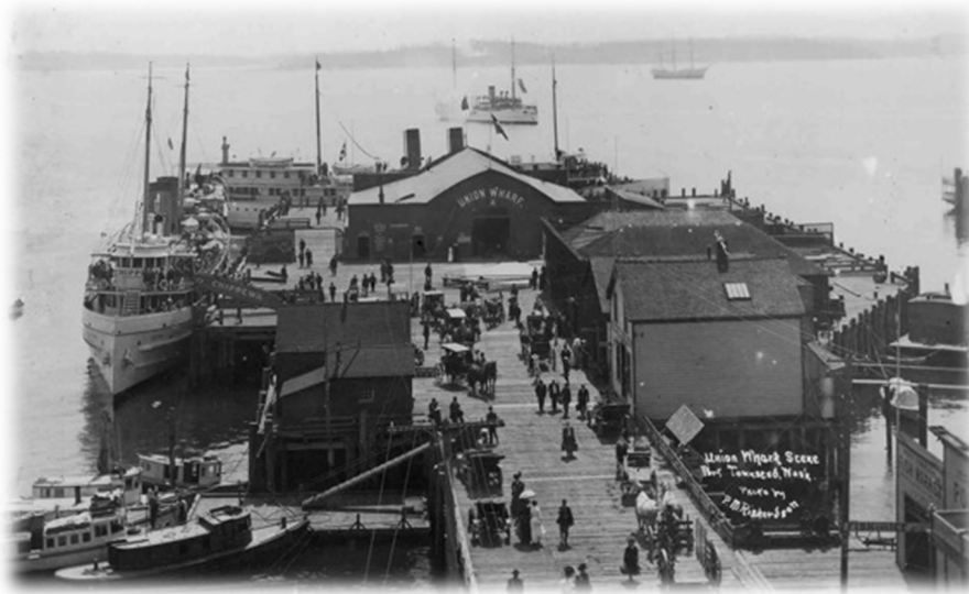
Old Union Wharf – Port Townsend, WA
