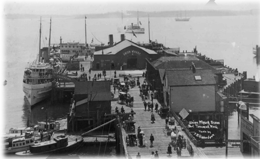
Old Union Wharf – Port Townsend, WA
