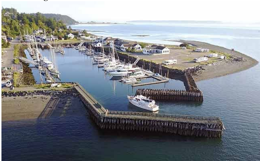
Figure III-4 - Aerial View – Point Hudson Marina & RV Park
