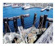
The project involves the total demolition and replacement of the Point Hudson Jetty. The jetty structure, built in 1934, has reached the end of its useful life and is at high risk of catastrophic failure if not replaced. Replacement of the breakwater ensures that the public's substantial existing investment in the Point Hudson Marina remains intact and ready to serve the public. Design and permitting will continue in 2017; construction is now scheduled to begin in 2018.
