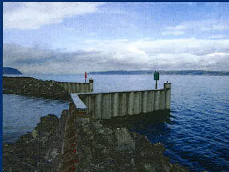
VERTICAL PILE (VP) BREAKWATER
