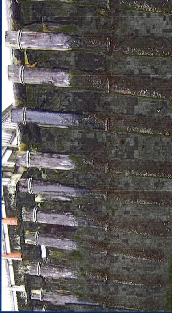
Piles in Poor Condition
