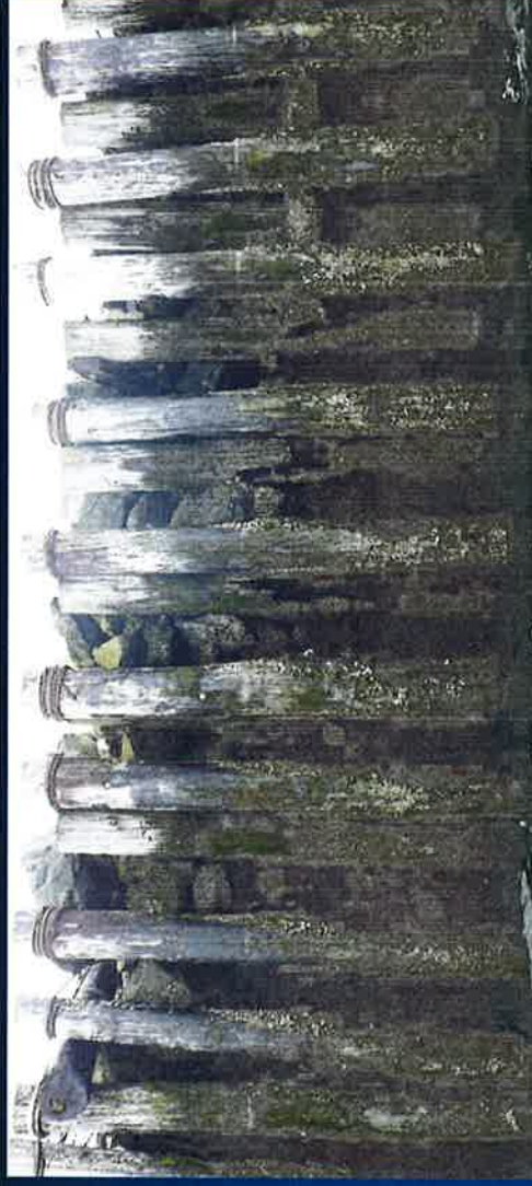
Piles in Poor Condition
