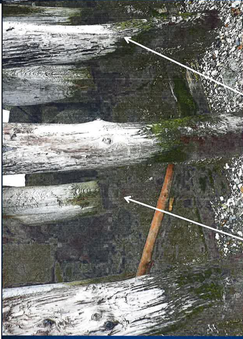
Inner Pile (1934) Abraded & Decayed
