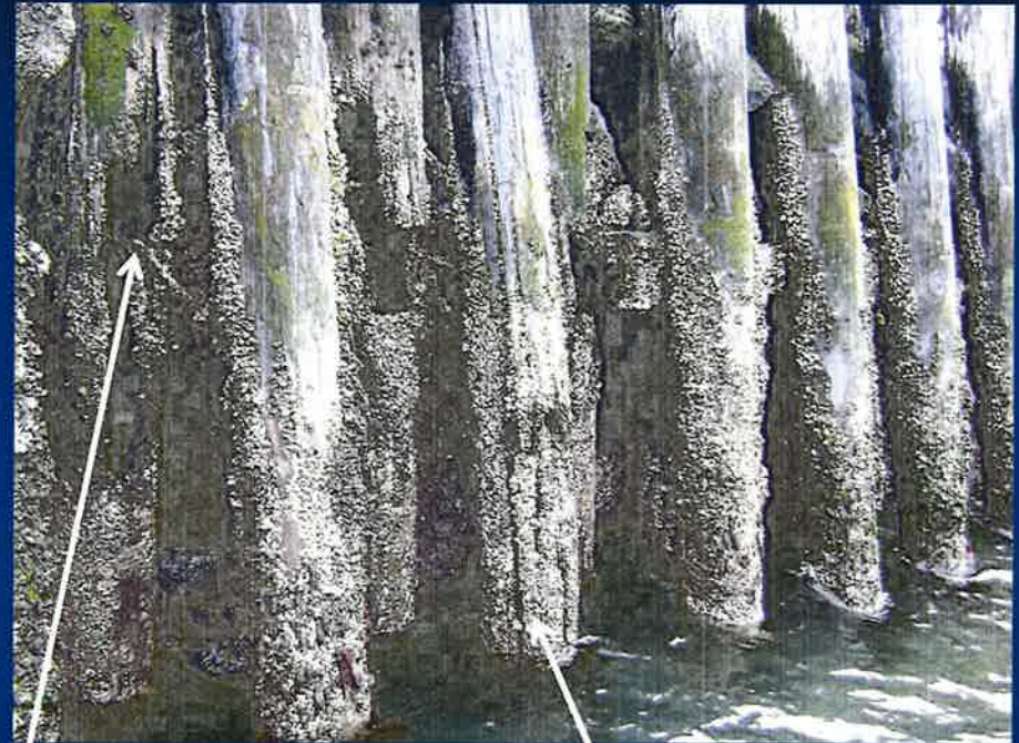
Outer Pile (1969): Marine Borer Attack
