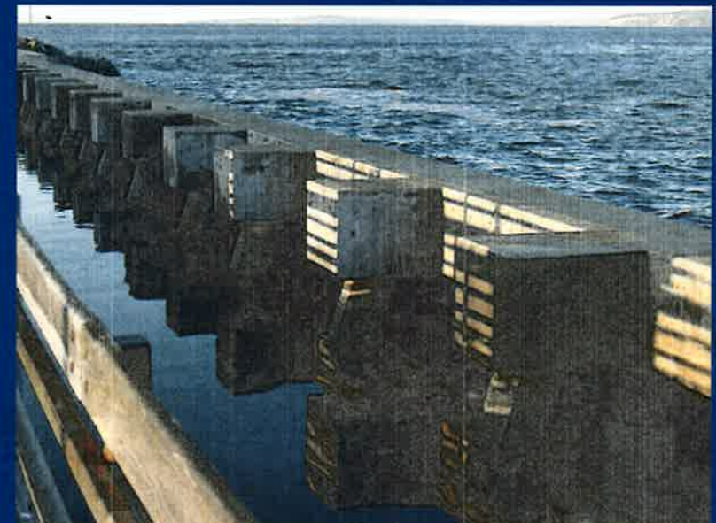
BRACED PILE (BP) BREAKWATER
