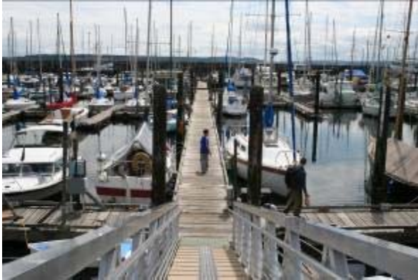
An overview of A/B Dock
