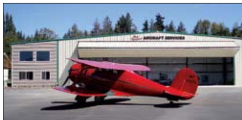
PT Aircraft Services' hangar was rebuilt and refurbished after an accidental fire in May 2008.
