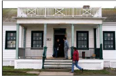
T's Restaurant will soon be moving into the Nurses' Quarters at Point Hudson. The Port has invested $175,000 into a historically sensitive remodel.
